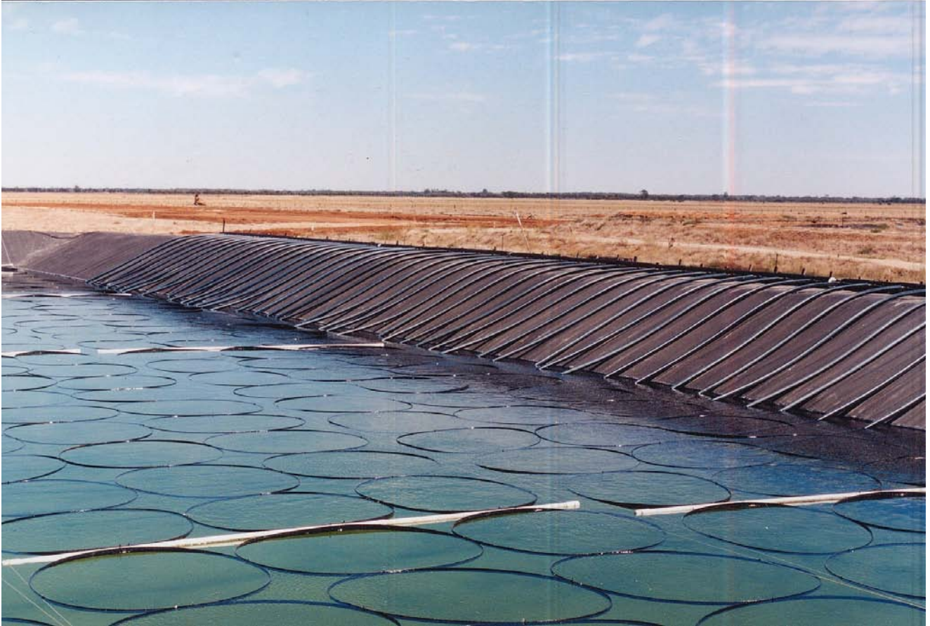
An example of a pilot solar pond, Pyramid Hill, Victoria (Photo: courtesy of Enersalt Pty Ltd)
