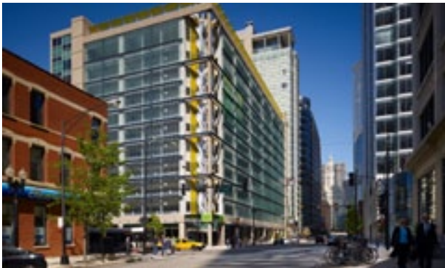
Facade-integrated wind turbines in Chicago, USA (Image: HOK and Steve Hall)
