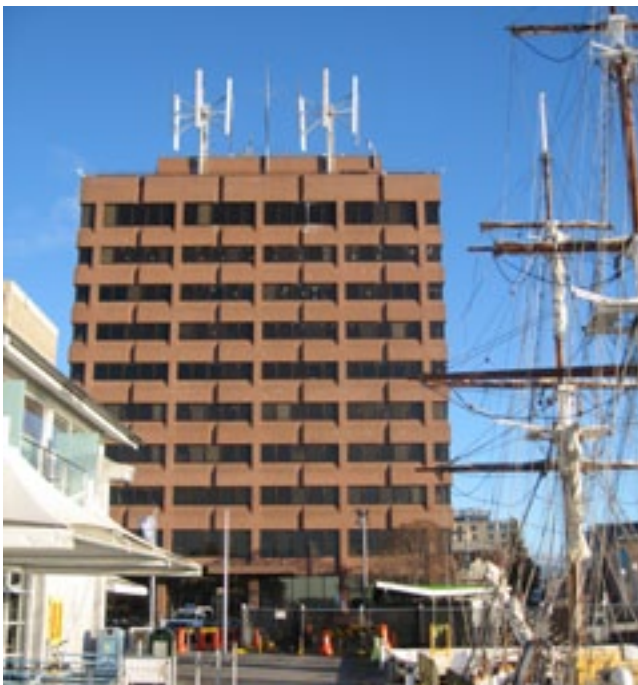
Wind turbines atop the Hobart Marine Board Building (Image: Xsquared Architects Pty Ltd, 2010)
