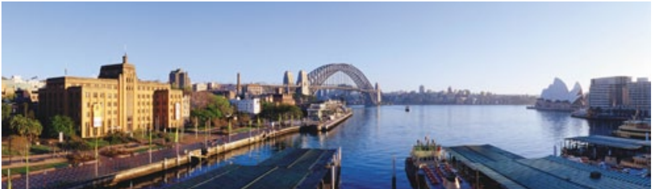
Museum of Contemporary Art will be cooled by Sydney Harbour (Image: MCA, 2010)
